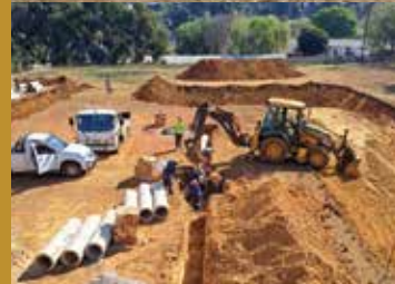
4. Civils under way
